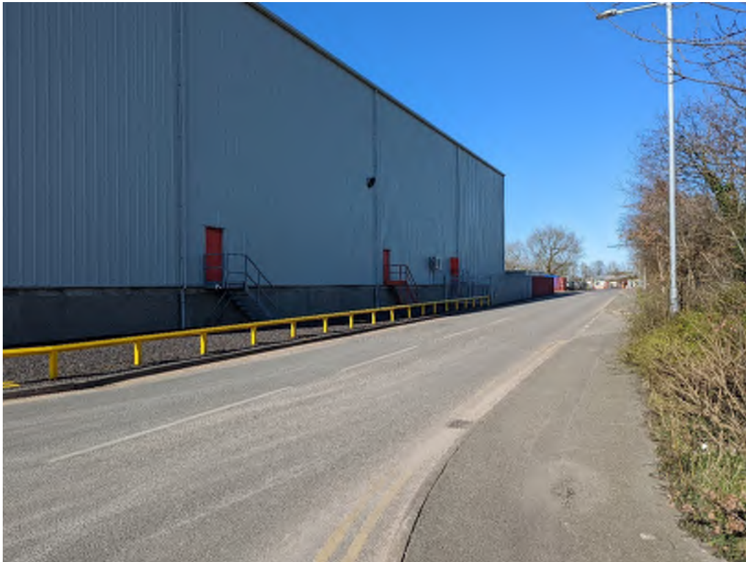
Photograph 19 – Eastern extent of warehouse at skip yard
