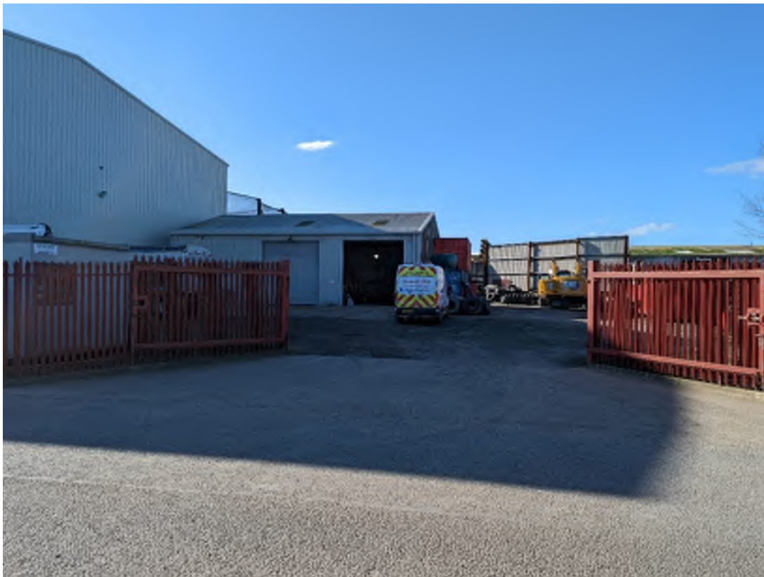
Photograph 20 – North eastern access to skip yard
