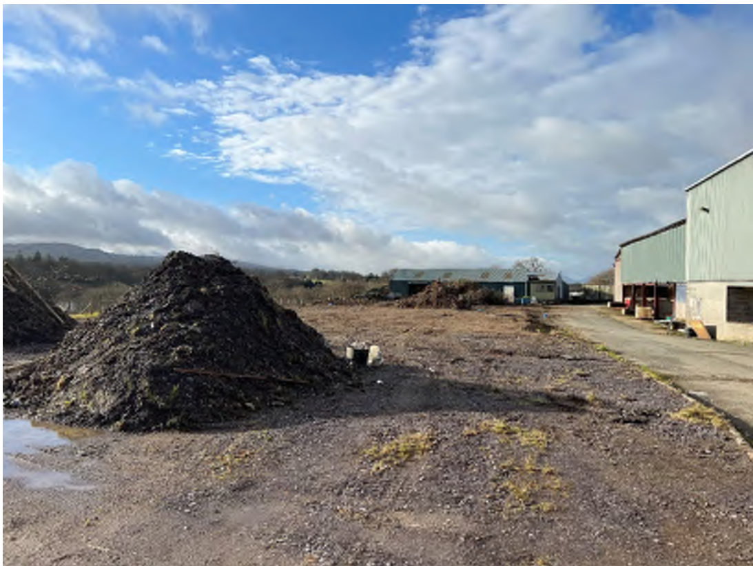
Photograph 6 – Stockpile of recently stripped topsoil at abattoir
