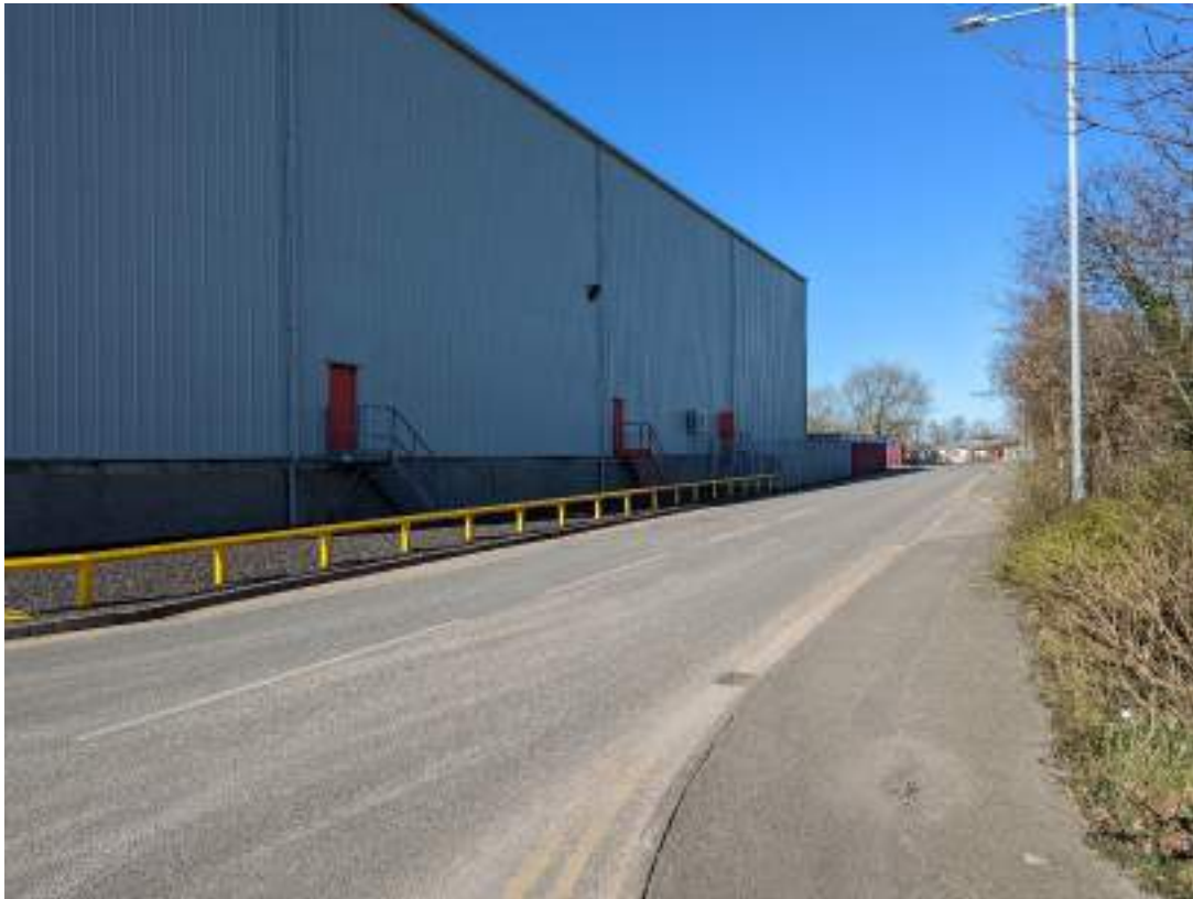
Photograph 19 – Eastern extent of warehouse at skip yard
