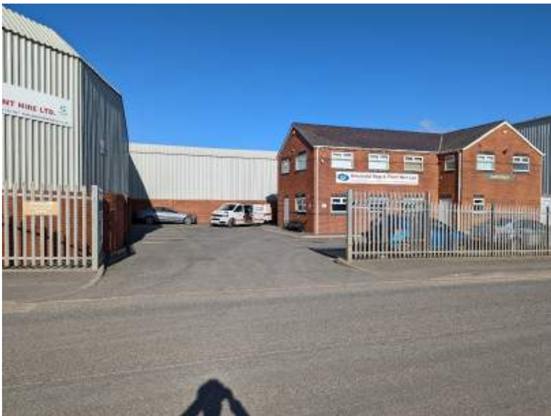
Photograph 18 – Site offices and cafe
