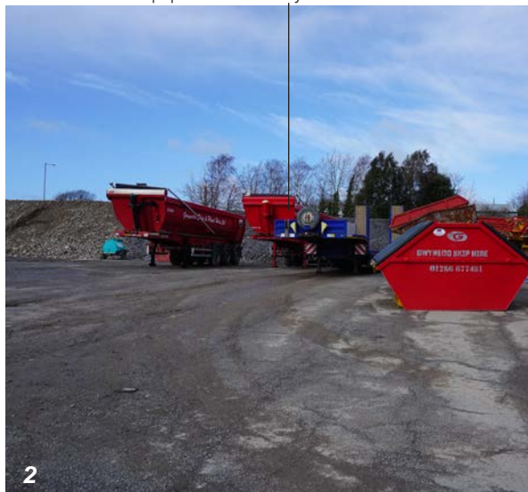
Mounds of rubble and large skips/ equipment currently on site
